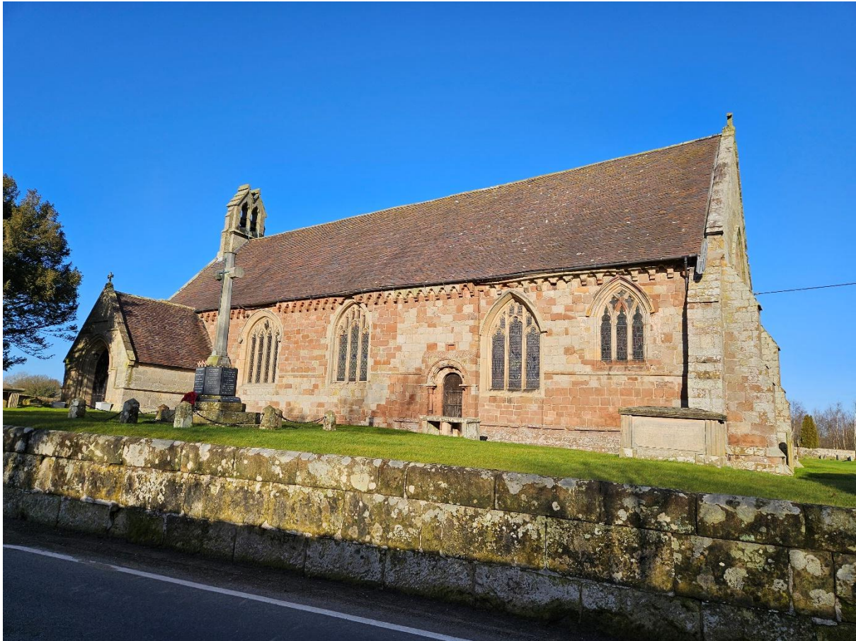
Figure 1. Edstaston church from the south, 2024 Photo: Wendy Horton for VCH Shropshire
